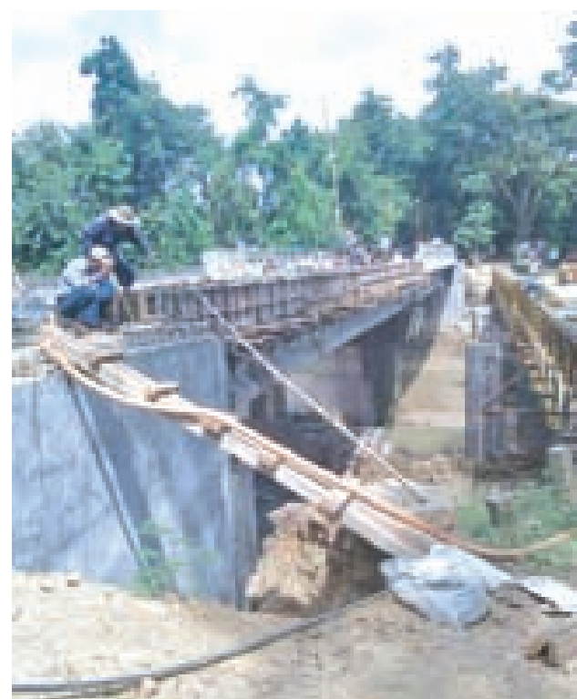
Pandawpyin Bridge is under construction on Thayet-Minhla-Minbu Road.
