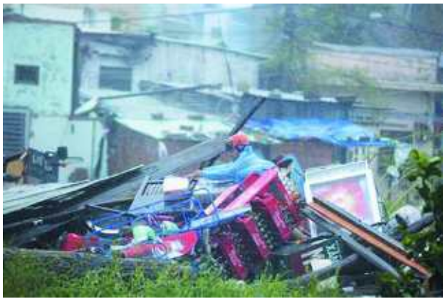
A man sorts through the remains of his home, which collapsed because of Typhoon Nari, in Vietnam's central Danang city, on 15 Oct, 2013.—REUTERS
