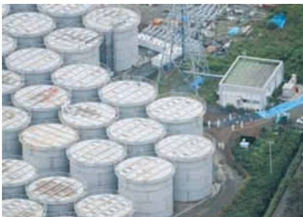
An aerial view shows workers wearing protective suits and masks working atop contaminated water storage tanks at Tokyo Electric Power Co.—KYODO NEWS
