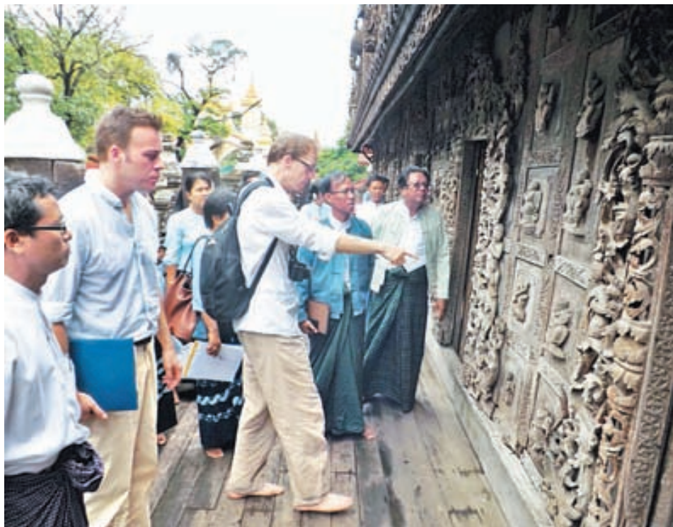
the Shwekyauungyi. They then observed damages of the building. Kyemon-Kyaw Htoo
