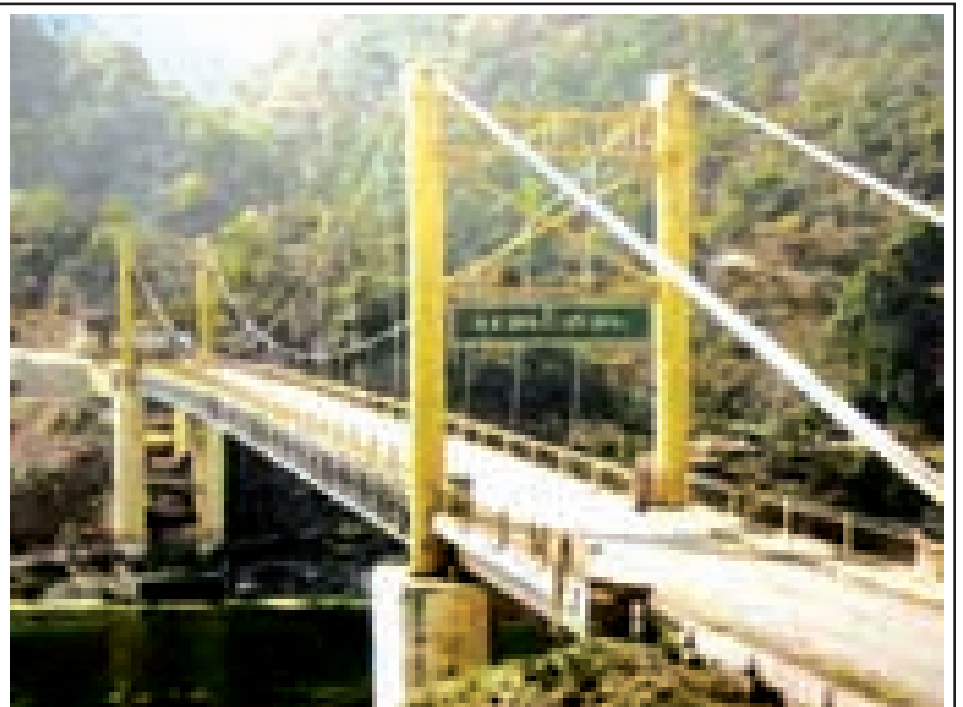
Photo shows Mansaung Bridge on Tiddim-Reed Lake Road in Chin State.
