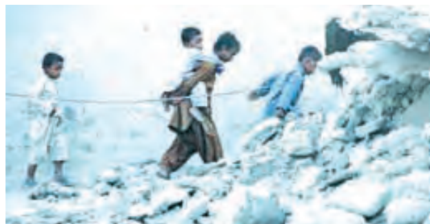
Survivors of an earthquake walk on rubble of a mud house after it collapsed following the quake in the town of Awaran, southwestern Pakistani province of Baluchistan, on 25 Sept, 2013.—REUTERS
