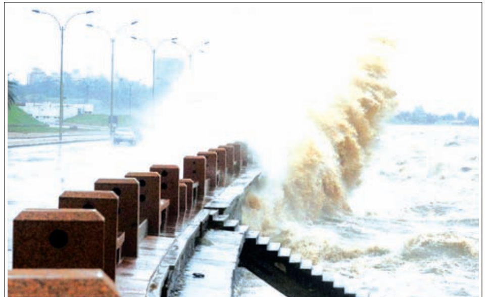
A wave hits the dam on the coastal avenue in front of the Rio de la Plata during the passage of the extra-tropical cyclone that affects the country, in Montevideo, capital of Uruguay, on 17 Sept, 2013. The Uruguayan authorities issued an orange alert for the next hours by the passage of extra-tropical cyclone that has already caused power shortage to more than 3,000 homes, and more than 600 people have been evacuated in various departments of the country.—XINHUA
