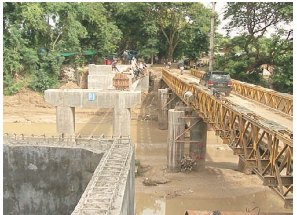
Photo shows a bridge under construction in Magway Region.—MNA
