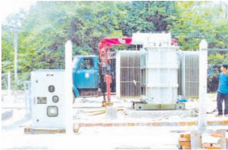
Photo shows the site of installation of new transformer in Ayadaw.
