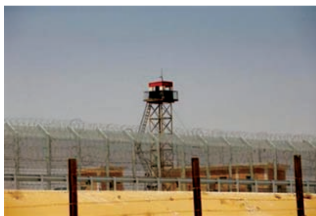
An observation tower painted in the colours of the Egyptian national flag is seen near the Nitzana crossing, along Israel's border with Egypt's Sinai desert on 20 Aug, 2013.—REUTERS
