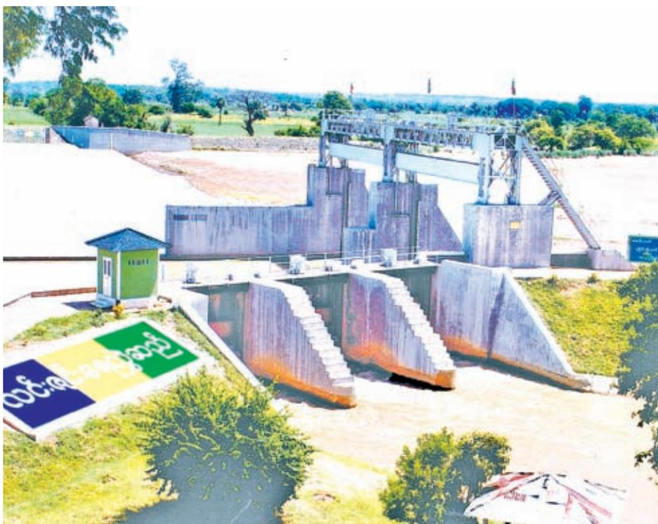
Linzin Diversion Weir and irrigation system were built in 1927 on Salin Creek near Linzin Village of Salin Township in Magway Region. Diversion weir, 750 feet long and seven feet high, is of concrete work. It has two 60x7.5 square feet sand sluice gates and three valves in 20x4.5 square feet size each.
