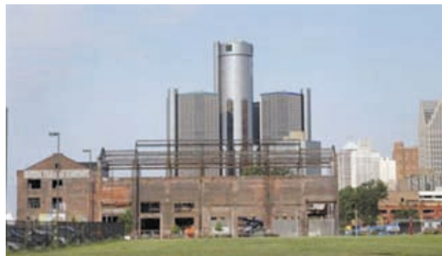
General Motors World Headquarters is seen behind a historic warehouse being restored along the Detroit River in Detroit, Michigan on 21 July, 2013.—REUTERS
