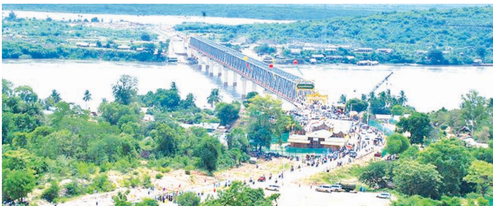
A bird eye's view of the newly opened Ayeyawady Bridge (Yadana Theinga).—MNA
