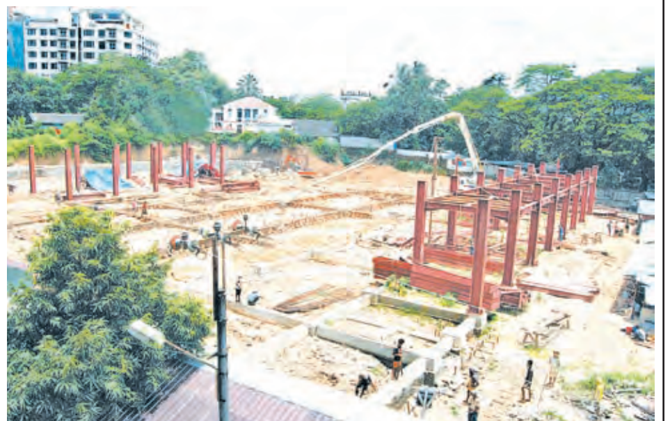
Construction of new market complex under way.—TIN SOE (MYANMA ALINN)
