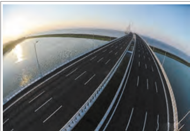
Photo taken on 17 July, 2013 shows the completed Jiashao Bridge which connects Jiaxing and Shaoxing in east China's Zhejiang Province. As the second cross-sea bridge spanning across the Hangzhou Bay, the Jiashao Bridge will be officially opened to traffic on 19 July. It will halve the travel time from Shaoxing to east China's Shanghai. —XINHUA
