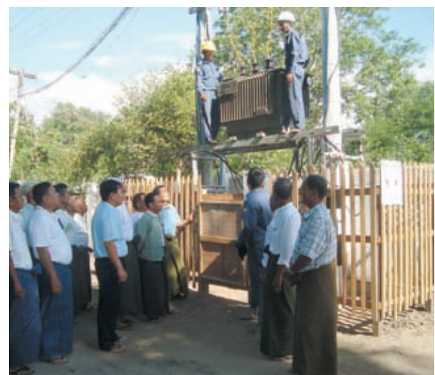
Electricians carrying out maintenance of transformer in Meiktila.
