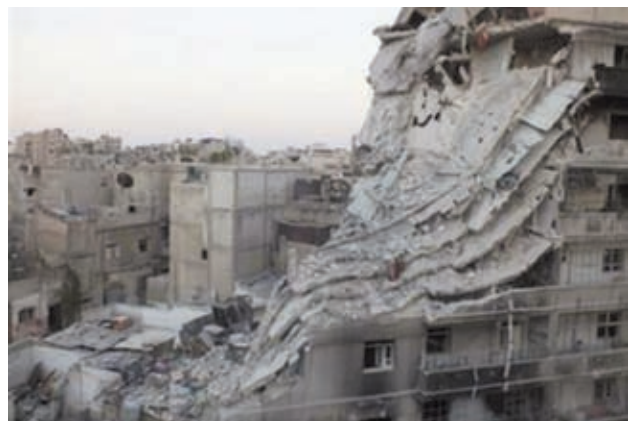
A general view shows buildings damaged by what activists said was shelling by forces loyal to Syria's President Bashar al-Assad in the Al-Khalidiya neighbourhood of Homs on 28 June, 2013.—REUTERS
