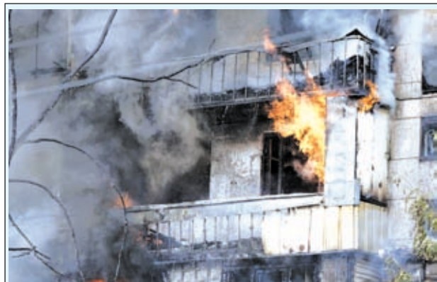
A building is flamed by a nearby explosion of a tanker in Almaty, Kazakhstan, on 27 June, 2013. A tanker turned over in Almaty on Thursday and then a blast and a fire occurred, making a nearby eight-storey building on fire, causing the tanker driver dead and over 20 residential buildings and about ten vehicles damaged.—XINHUA
