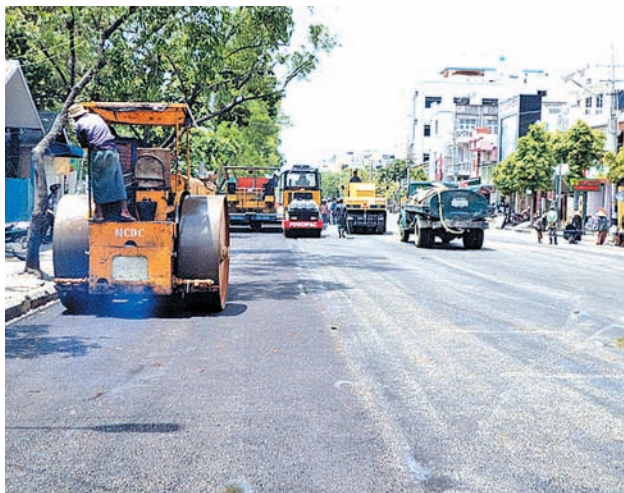
Road to Mandalay University being upgraded with the use of roller.
