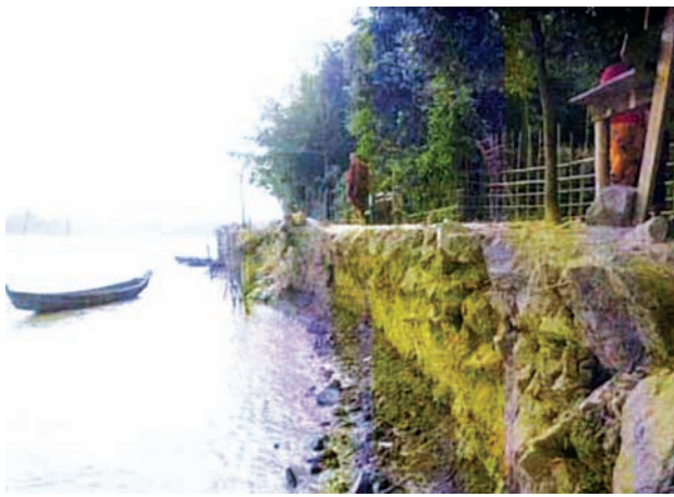
WAW, 8 June—The bank of Sittoung River are facing landslides due to
