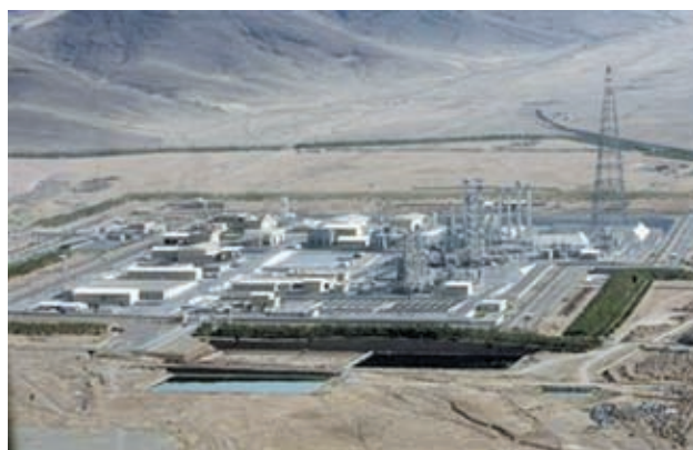
A view of the Arak heavy-water project 190 km (120 miles) southwest of Teheran on 26 Aug, 2006. Iran President Mahmoud Ahmadinejad launched a new phase in the Arak heavy-water reactor project on Saturday, despite Western fears it is aimed at producing a bomb.—REUTERS
