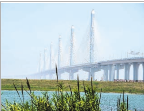
The construction of the main towers of the Jiaxing-Shaoxing Sea-crossing Bridge is finished in Shaoxing, east China’s Zhejiang Province, on 24 May, 2013. The bridge is expected to be open to traffic by the end of June this year. It will halve the driving time from Shaoxing to Shanghai in east China after it is finished.—XINHUA
