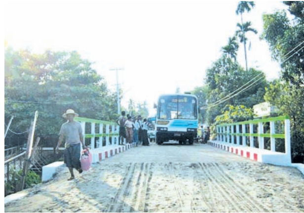
Photo shows newly-built Kyaiklat Pagoda Creek Bridge.
