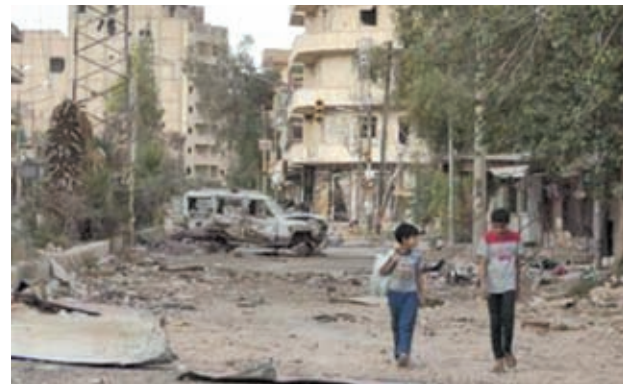
Boys walk along a damaged street filled with debris in Deir al-Zor on 19 May, 2013.—REUTERS
