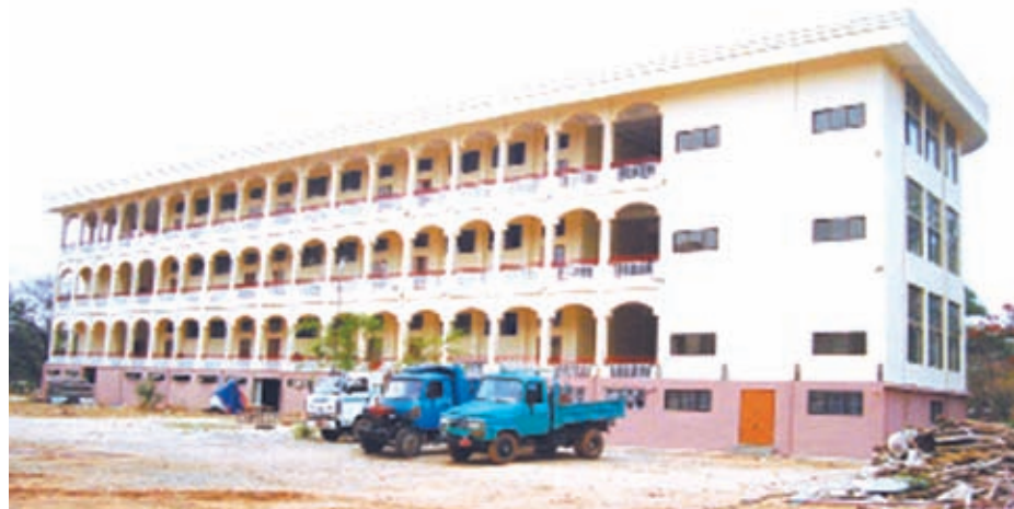
The newly constructed three-storey building in Meiktila University Campus.
