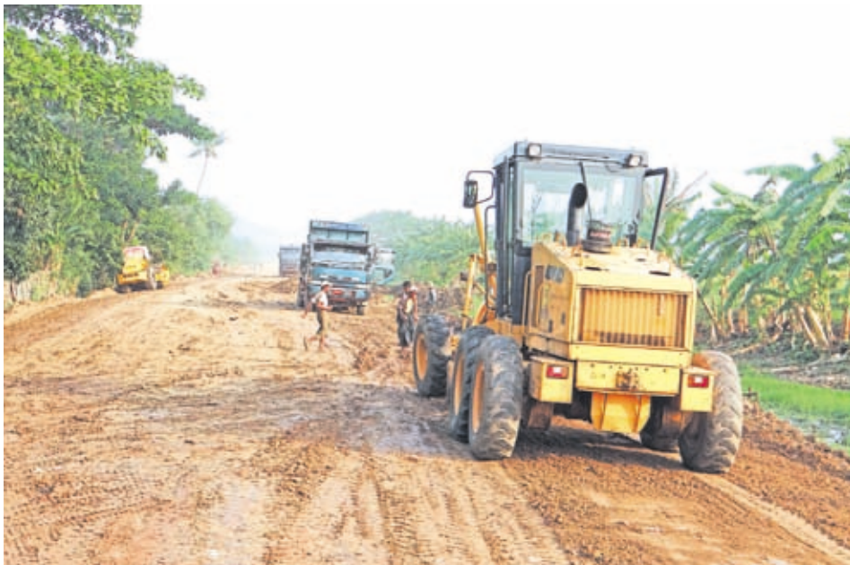
Road construction work seen with heavy machinery.—MNA
