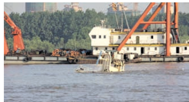
Photo taken on 12 May, 2013 shows the water area where a cargo vessel sank near the Nanjing Yangtze River Bridge in Nanjing, capital of east China's Jiangsu Province. The vessel, loaded with 12,500 tons of limestone, sank after rubbing against a pier of the bridge on Sunday. A total of 18 sailors on board were all saved.—XINHUA
