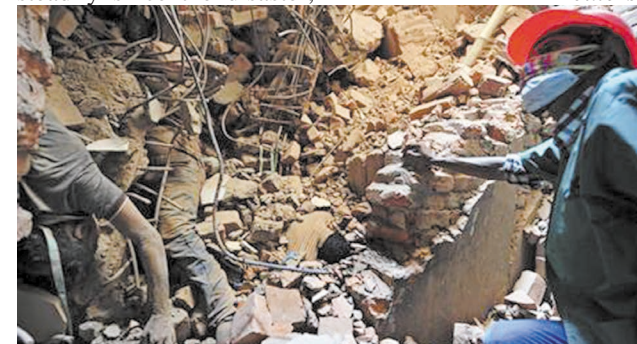
A rescue worker is seen next to the bodies of garment workers lying among the rubble of the collapsed Rana Plaza building, in Savar, 30 km (19 miles) outside Dhaka on 25 April, 2013.—REUTERS
