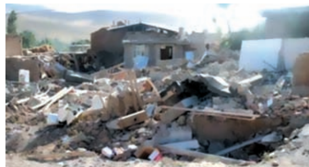
Damaged houses are seen in the earthquake stricken town of Bushehr in Iran on 9 April, 2013.—REUTERS
