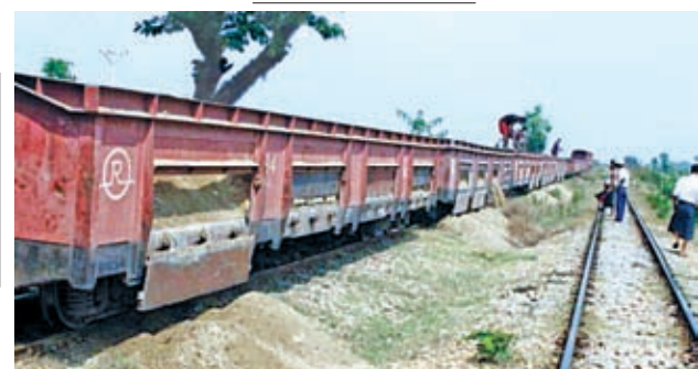
Photo shows stockpiles of stones and sand along Yangon-Mandalay railroad where maintenance works for safety of trains were carried out on 28 March.
