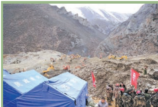
Rescuers work at the accident site in Maizhokunggar County of Lhasa, southwest China’s Tibet Autonomous Region, on 31 March, 2013. Thirteen bodies have been found until 6:30 pm on Sunday at the site of a mining area landslide. The disaster struck a workers’ camp of the Jiama Copper Polymetallic Mine at about 6 am on Friday, burying 83 workers. XINHUA
