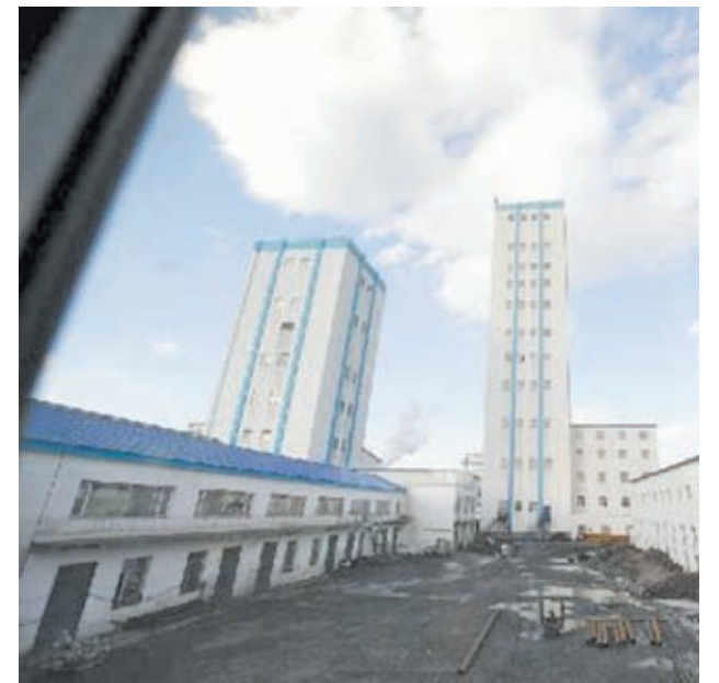
Photo taken on 30 March, 2013 shows the exterior where a gas blast happened at Babao Coal Mine in Jiangyuan District in the city of Baishan, northeast China's Jilin Province. Twenty-eight people were confirmed dead and 13 others injured during the colliery gas blast which happened around 10:40 pm (1440 GMT) on 29 March. The injuries of the 13 were not life threatening, said a spokesman with the provincial work safety and supervision bureau. Rescue work has been finished, and the cause of the accident is under investigation.—XINHUA
