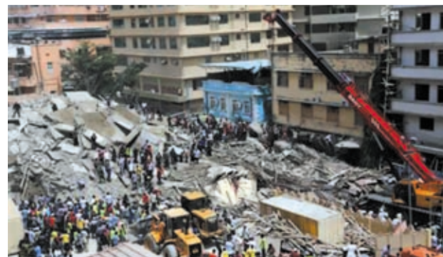
An aerial view shows bystanders watching rescuers search for survivors amongst the rubble of a collapsed building in the Kariakoo District of central Dares Salaam on 29 March, 2013.—REUTERS
