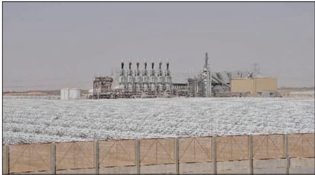
Photo taken on 17 March, 2013 shows the newly launched solar plant Shams 1 in the desert of Abu Dhabi, the United Arab Emirates.—XINHUA
