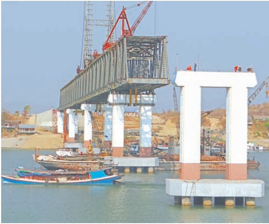
Construction of Ayeyawady Bridge (Malun) in progress.—MNA
