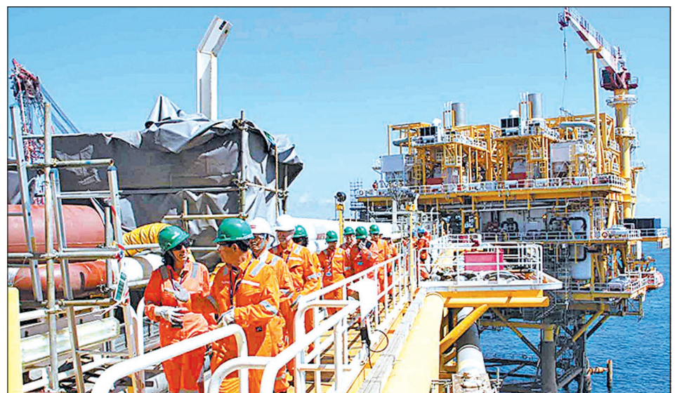
Union Minister for Energy U Than Htay views production platform of Yadana gas field project in the Gulf of Mottama.—MNA
