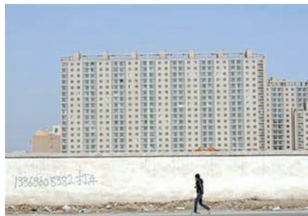
A man walks past a wall at a construction site at a new residential area in Beijing on 27 Feb, 2013. REUTERS
