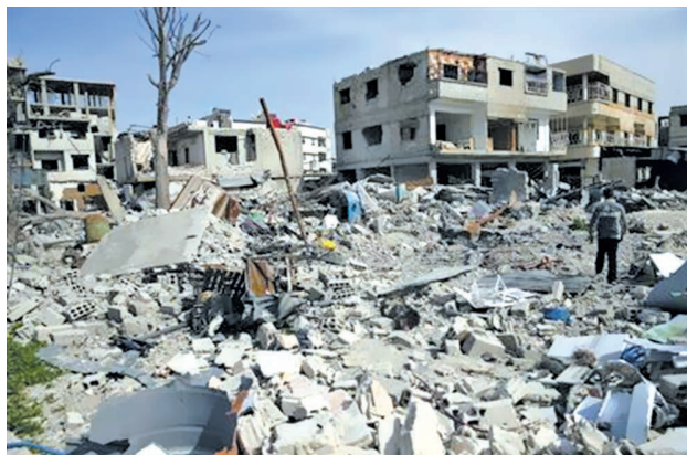
A man walks at the damaged Harasta area that was caused by forces loyal to Syrian President Bashar al-Assad, in Damascus on 25 Feb, 2013.—REUTERS
