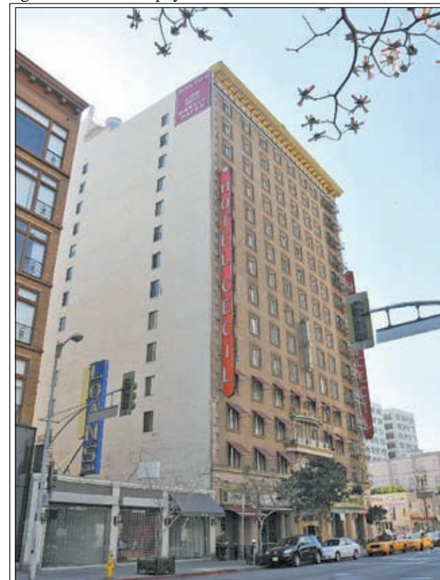
Photo taken on 23 Feb, 2013 shows Cecil Hotel where a girl was found dead on Tuesday, in Los Angeles, the United States. Cecil Hotel closed on Saturday for repairing of water pipes and will reopen next Tuesday. The body of Elisa Lam from Vancouver was found on Tuesday in a water cistern atop the downtown Cecil Hotel.—XINHUA
