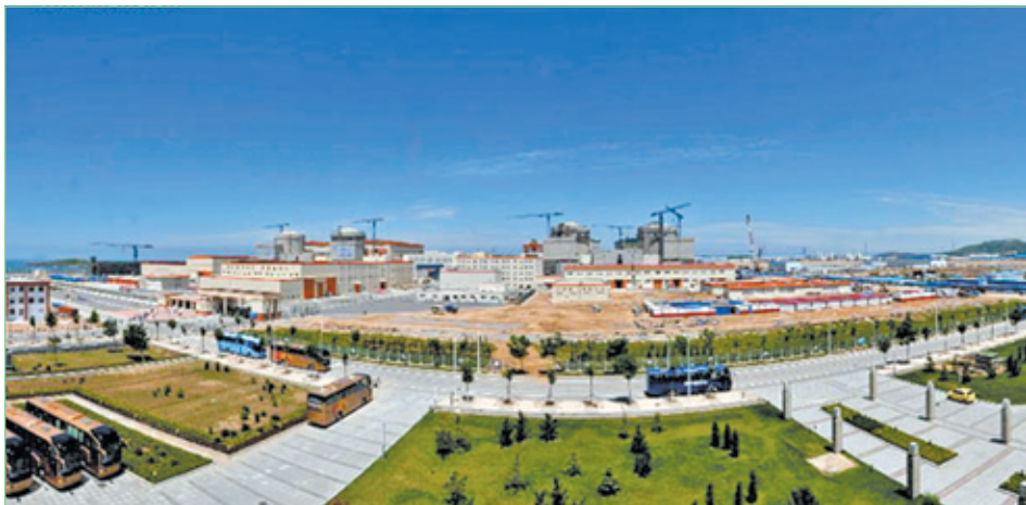
Photo taken on 12 July, 2012 shows the Hongyanhe nuclear power station near Wafangdian, northeast China's Liaoning Province. The Hongyanhe nuclear power station, the first nuclear power plant and largest energy project in northeast China, started operation on Sunday afternoon.—XINHUA
