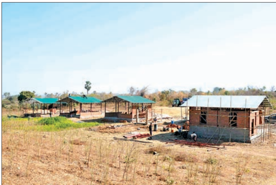
Photo shows progress in construction of affordable houses.—MNA
