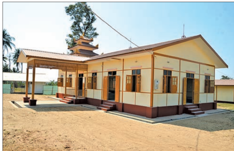
Photo shows a newly-built Dhammayon building in Shwekyarpin ward of Zabuthiri Township in Nay Pyi Taw Council Area. It was constructed by Nay Pyi Taw Development Affairs Committee that spent K 82.5 million on construction of the 72 feet long and 32 feet wide one-storey RC building. The building was handed over to the administrator of Shwekyarpin ward on 25 January. — MNA
