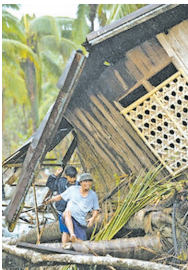
Rene Diano tries to collect nails and debris from his wrecked house in New Bataan town in Compostela Valley province in southeastern Mindanao in the Philippines on 2 Jan, 2013, about a month after typhoon Bopha devastated the area.
