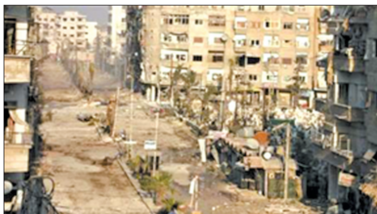
A view of buildings damaged by what activists said were missiles fired by a Syrian Air Force fighter jet loyal to President Bashar al-Assad in Daraya, near Damascus, on 29 Dec, 2012.
