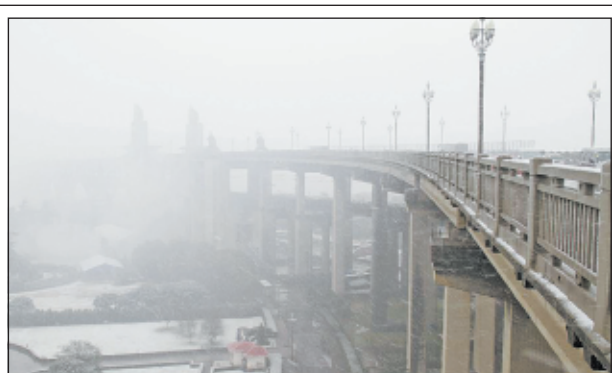
Photo taken on 29 Dec, 2012 shows the Nanjing Yangtze River Bridge in snow in Nanjing, capital of east China's Jiangsu Province. Nanjing witnessed a snowfall on Saturday, which also marked the 44th anniversary of the bridge's opening to traffic in 1968.—XINHUA
