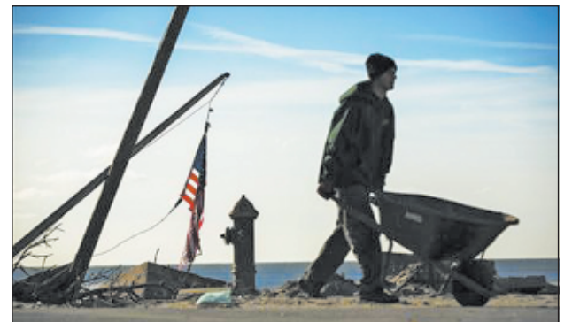
Contractor Chris Siller pushes a wheelbarrow full of sand to fill in a lawn damaged by superstorm Sandy two months after the storm caused extensive damage in the Queens borough region of Belle Harbour, New York, on 28 Dec, 2012.—REUTERS
