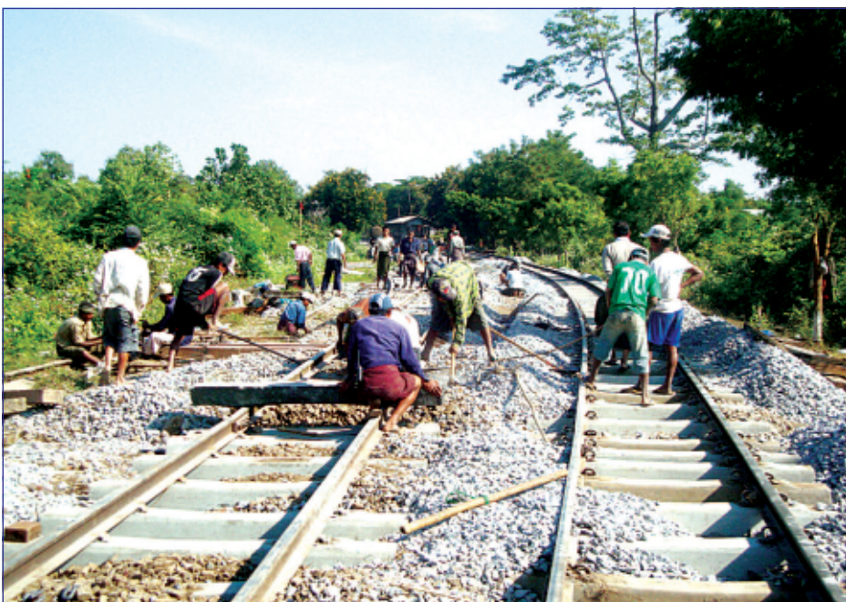
MR workers race to finish railroad repair faster than expected.
