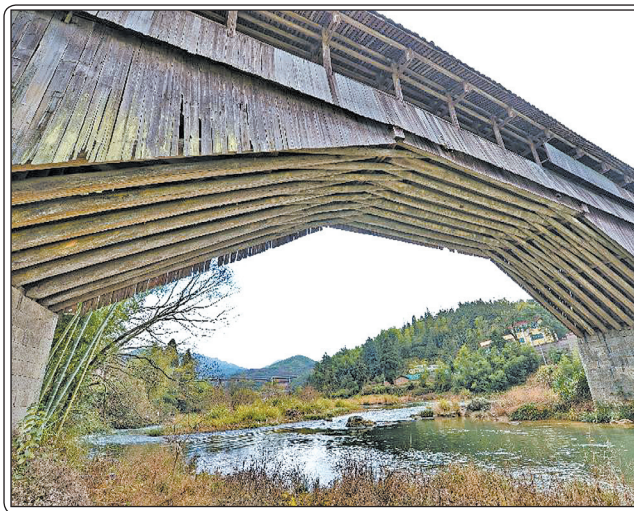
Qiancheng Bridge, a timber arch lounge bridge, is seen in Tangkou Village of Pingnan County, southeast China's Fujian Province, on 21 Dec, 2012. Built in the Southern Song Dynasty (1127-1279 AD) and rebuilt several times since then, the bridge is 62.7 metres long and 4.9 metres wide. It has been listed as one of the state key cultural relics protection units.—XINHUA
