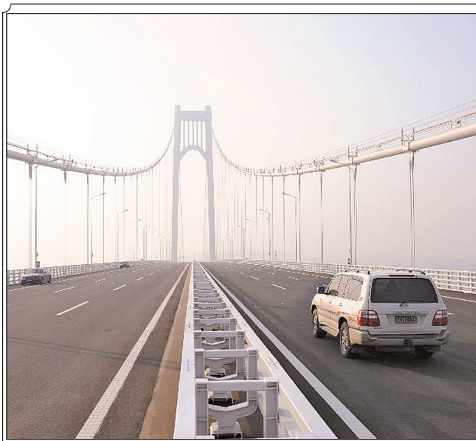
Vehicles run on the No 4 Nanjing Yangtze River Bridge in Nanjing, capital of east China's Jiangsu Province, on 24 Dec, 2012. The bridge was opened to traffic on Monday. The 28.966-kilometre-long suspension bridge supported by two towers and three spans, has a 1,418-metre-long main span, the longest among the same kind bridges in China and the third longest in the world.—XINHUA
