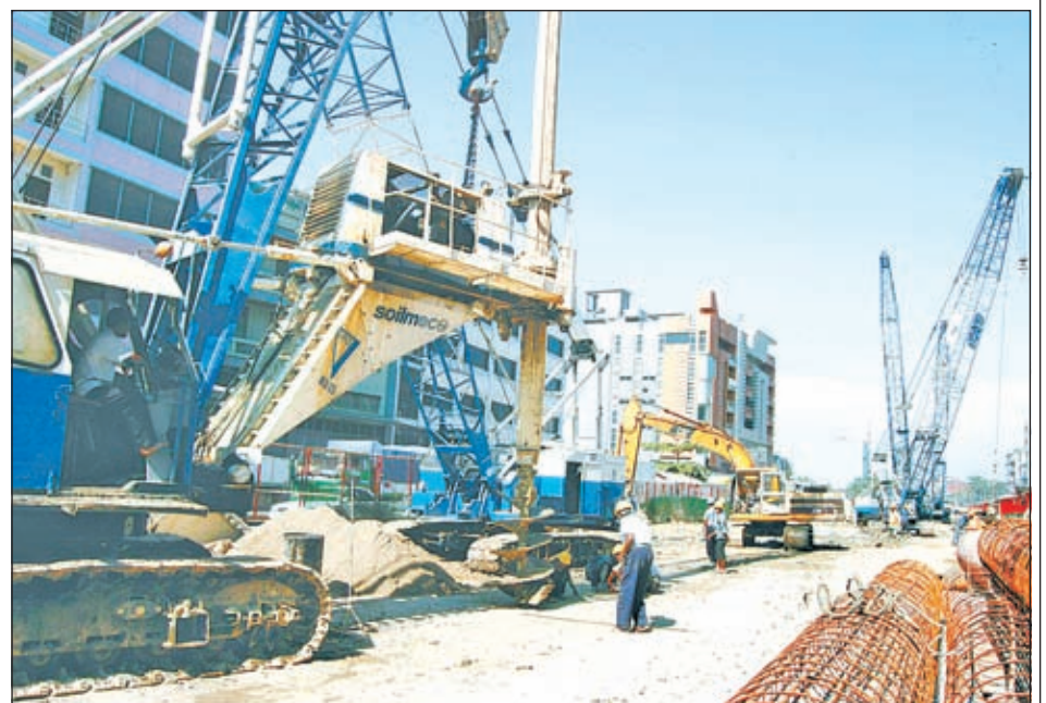
Bayintnaung Flyover is under construction with the use of heavy machinery.
