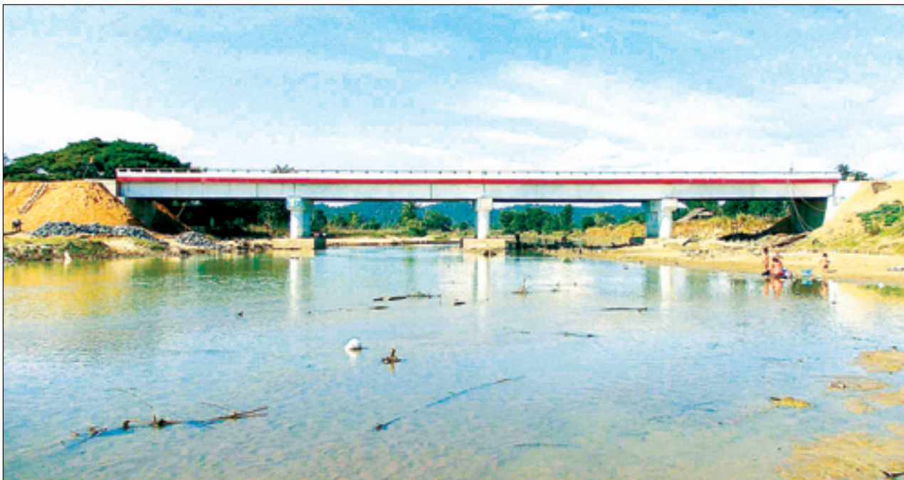
Tonsi Bridge, crossing the Namee Creek in Indaw Township of Sagaing Region.
