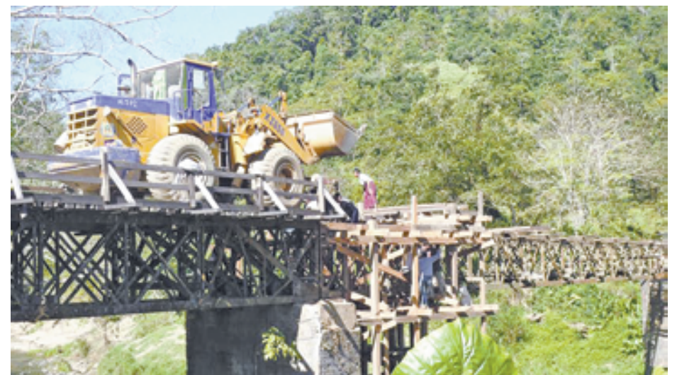
Construction of Insup Bridge on Myitkyina-Sumprabum-Putao Road in progress.
