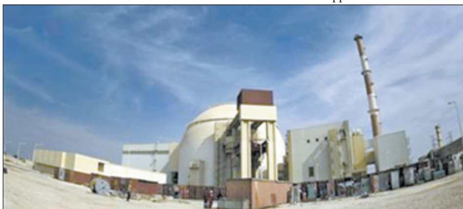
A general view of the Bushehr nuclear power plant, some 1,200 km (746 miles) south of Tehran on 26 October 2010. —Reuters
