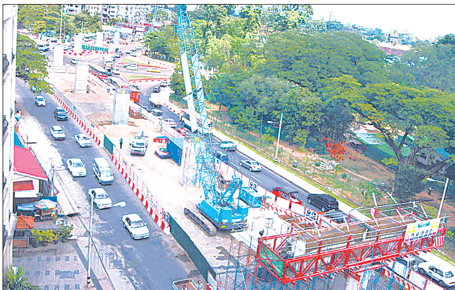
Hledan overpass construction in progress. Construction is completed by 65 percent.
